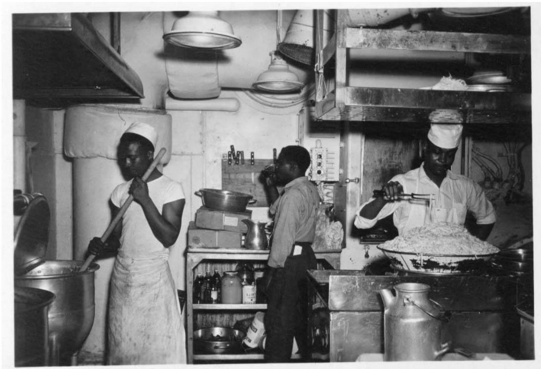
Men working in the Officer's Galley on board USS North Carolina , 1945
